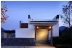
Household Energy Storage
