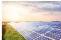
Energy Storage System
