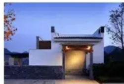
Household Energy Storage
